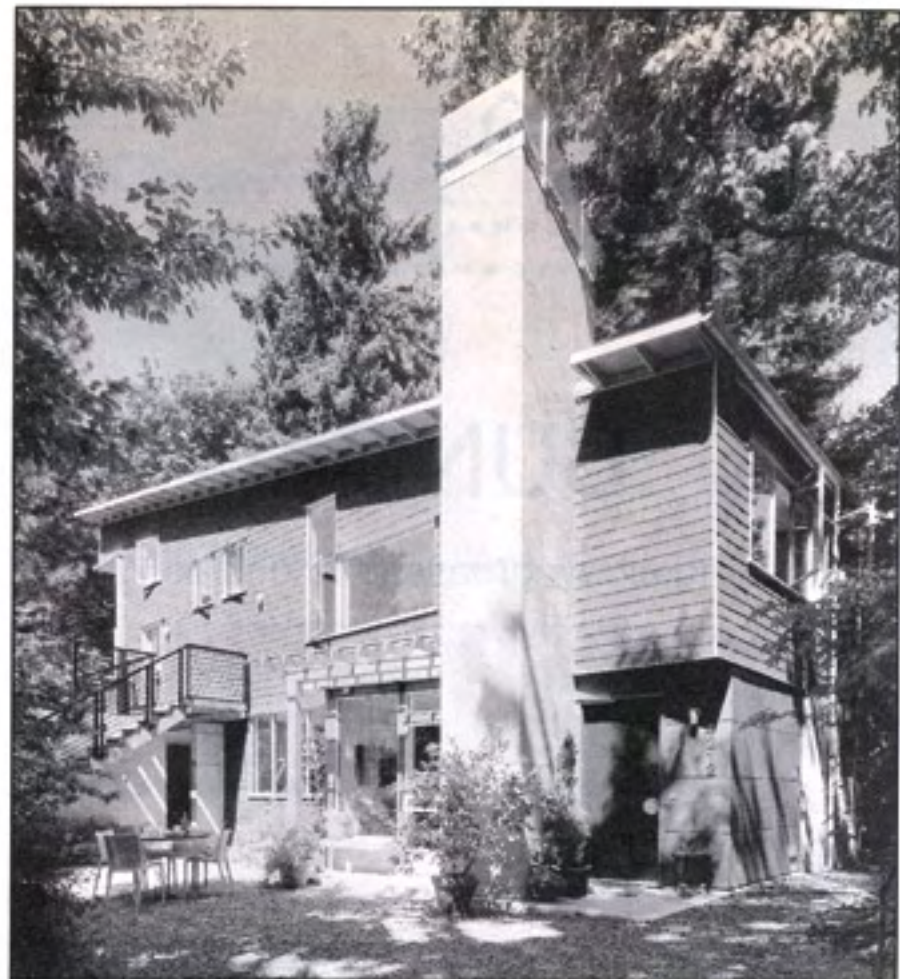
DESIGNED TO BE BUILT in stages, the home lacks the fourth courtyard "wall." When the budget allows, the front door (and corresponding side wall) will "wrap around" the chimney base (and add 300 square feet). To the far left, an exterior stairway leads to the stucco space.
